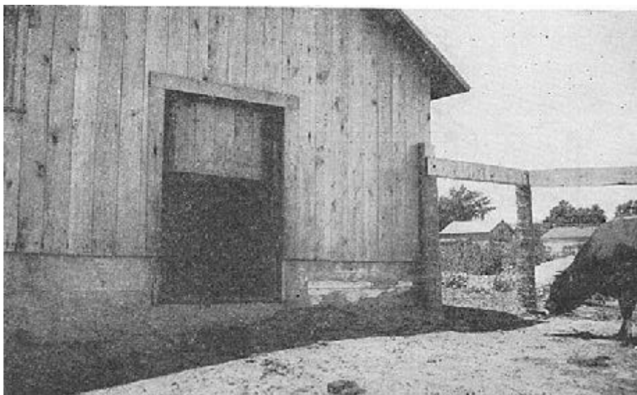
Fig. 9. A vertical-sliding door is not easily damaged by the bull.
